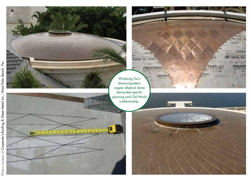
Each panel was anchored with four interlocking copper cleats and eight flat-head stainless-steel concrete fasteners—two fasteners per cleat. The fasteners were chosen because they are suitable for concrete, coppercompatible and the head will not telegraph to the roof's surface.
